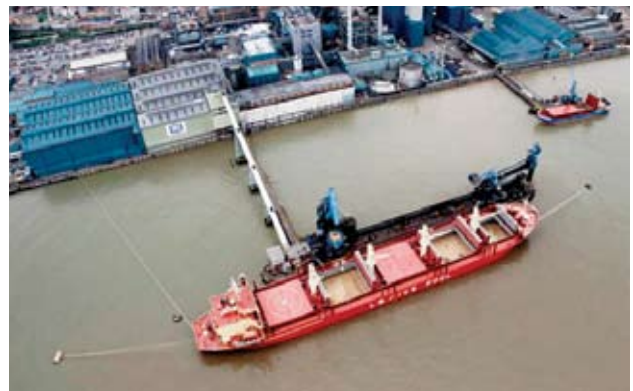
Tate & Lyle's Silvertown operation is one of the Port's longest standing customers, handling over one million tonnes of cane sugar a year
