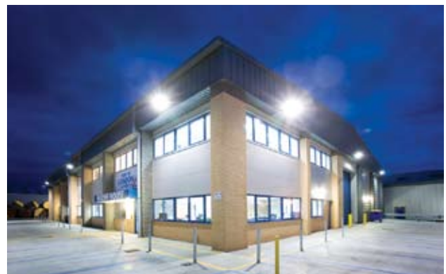
Marine House boasts environmental features including a rain water harvesting system and movement-activated lights
