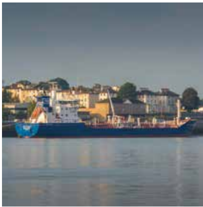
COMPLETED PROJECT WITH FM CONWAY TO BRING IMPERIAL WHARF, GRAVESEND, BACK INTO USE AS A BITUMEN TERMINAL
